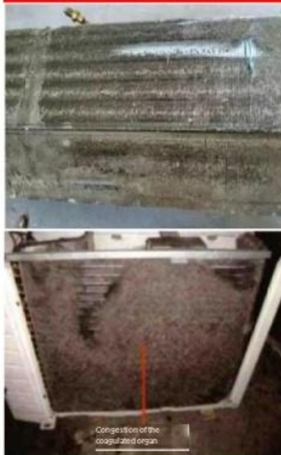
The heat exchanger surface is dirty and blocked
