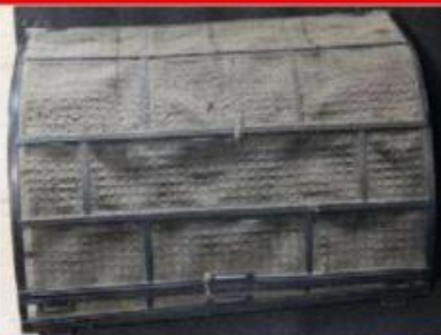
The heat exchanger surface is dirty and blocked
